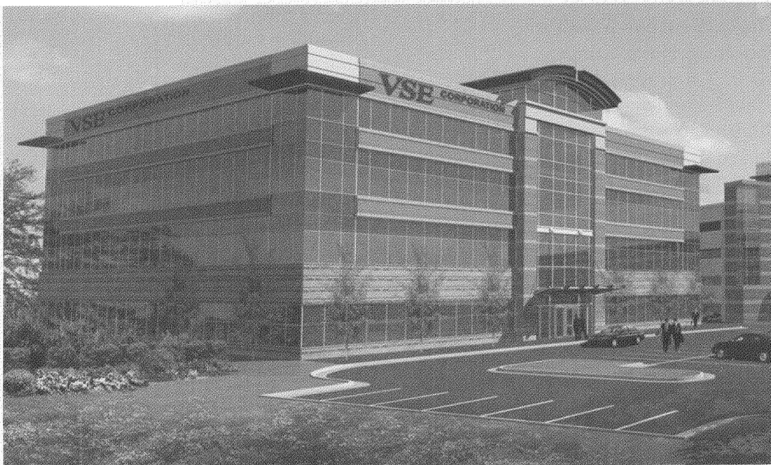
Artist rendition of new VSE Headquarters in Springfield, Virginia set to open in Spring 2012.
